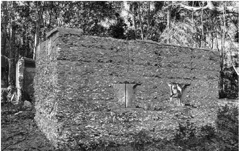
An early Gullah sugar works near Darien, Georgia, showing typical tabby construction in the Lowcountry of the nineteenth century, making walls from crushed oyster shells. (Courtesy of the National Park Service.)
